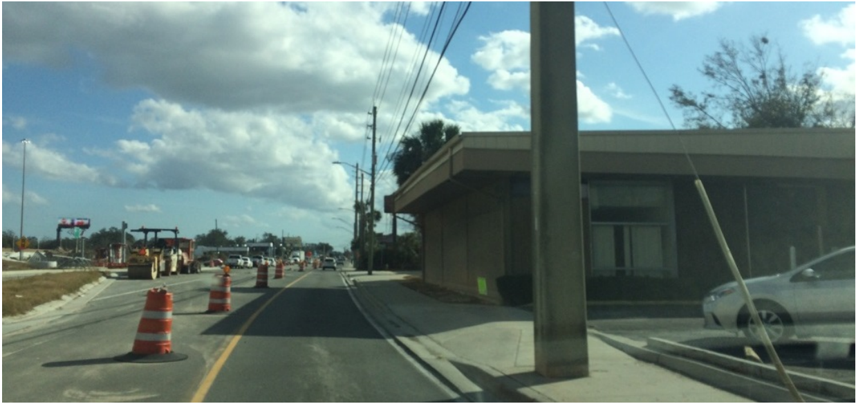
View of the subject property on the right facing south along Kings Ave/Philips Hwy
