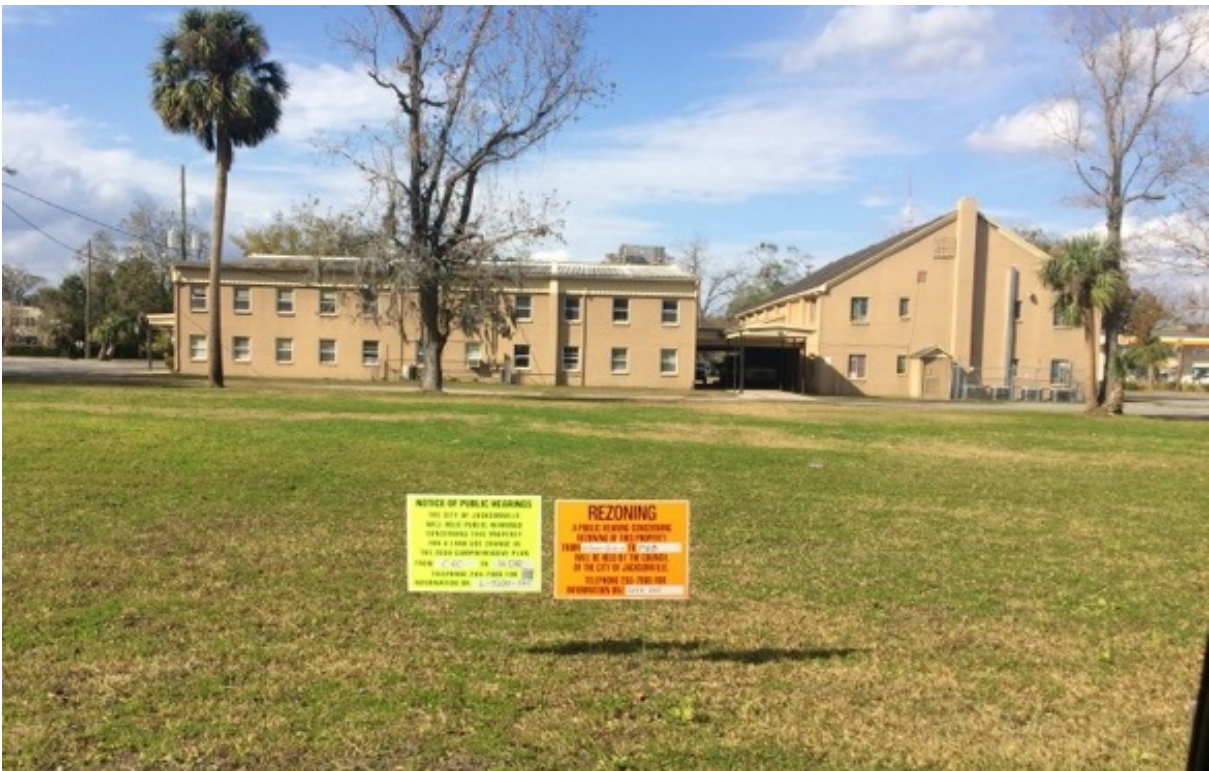
View of the subject property facing north from Mitchell Ave.
