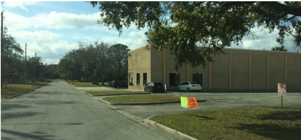
View of the subject property on the right facing west along Bertha St.
